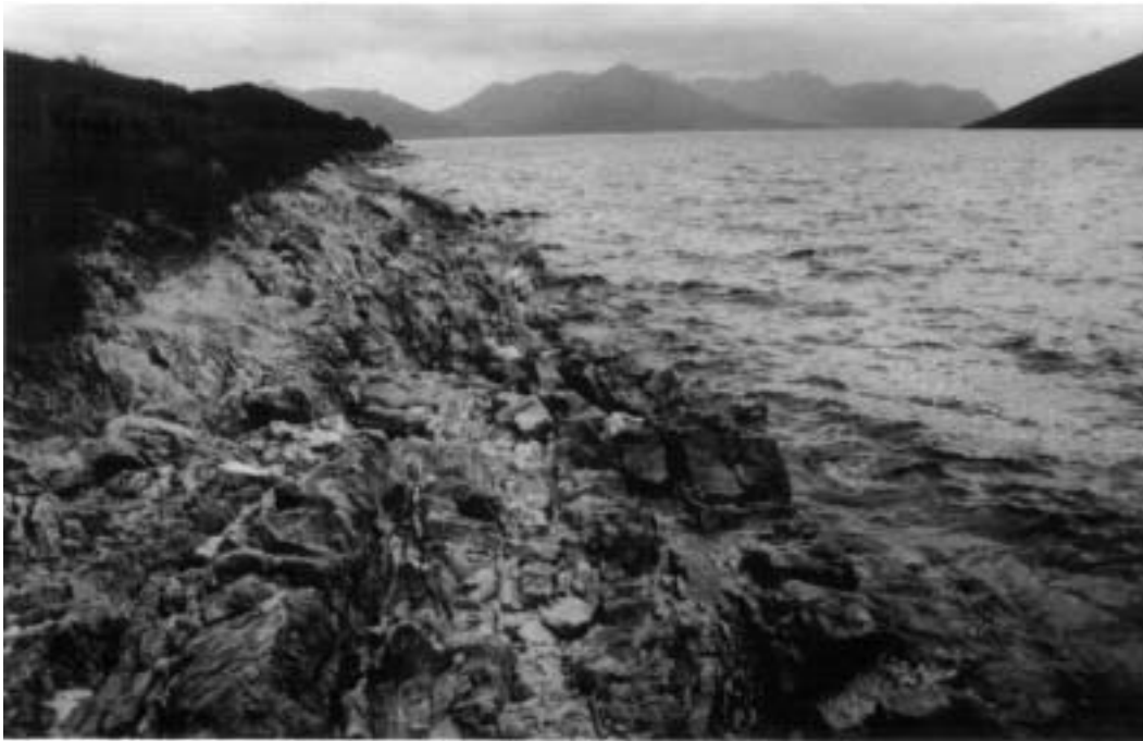
Figure 8c: Degree 4 damage. Stripping of shallow peat to expose a bedrock shore on a steep margin of the reservoir west of the Scotts Peak Dam exposed to the full fetch of the largest waves (photo: K. Kiernan).
