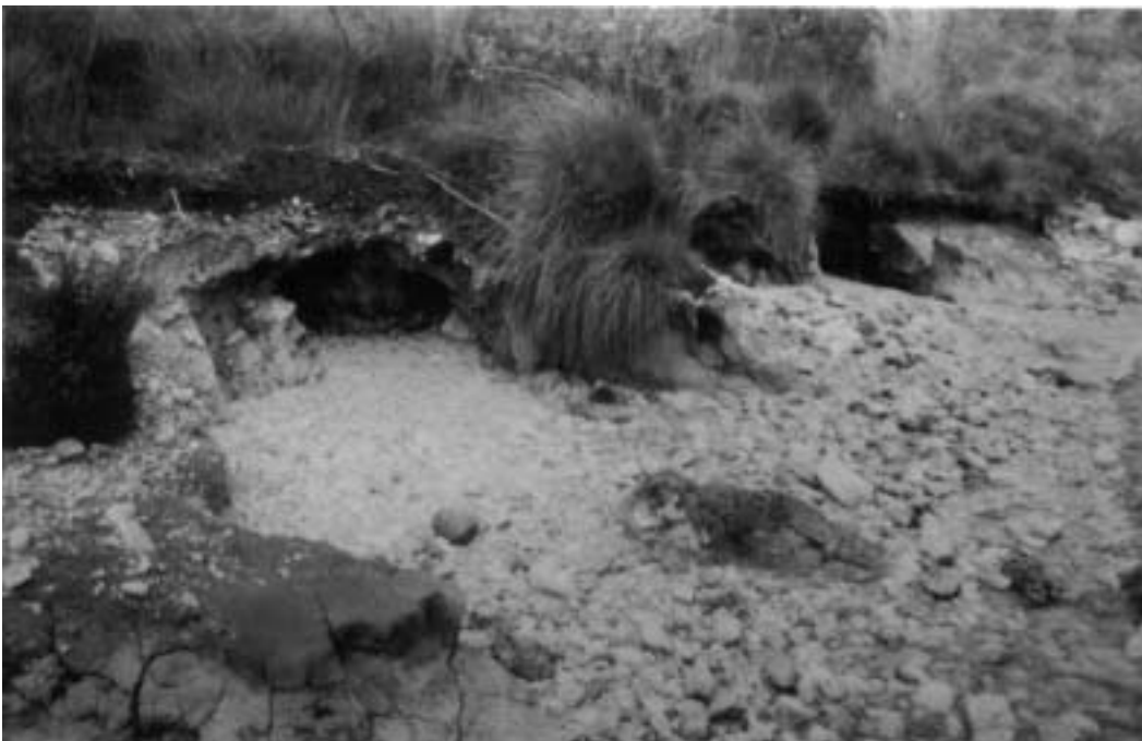
Figure 7c: Degree 3 damage. Cliffing of sandy regolith in embayments between remnant peat promontories (foreground). Minor tunnelling in loose regolith beneath peat at head of embayments (photo: K. Kiernan).
