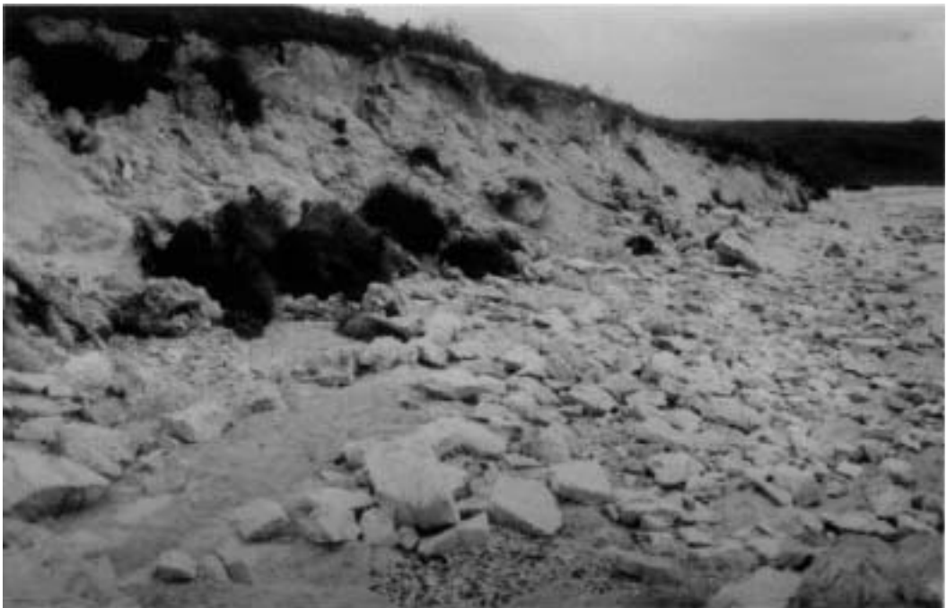
Figure 8b: Degree 4 damage. Scarp 2 - 3m high formed entirely in surficial sediments east of Scotts Peak Dam. This major cliffing is at the most severely eroded site identified during this survey, and is located at the exposed southern end of the reservoir. The blocks and cobbles in the foreground have been reworked from the regolith with the larger rocks piled towards the back of the beach by wave action (photo: K. Kiernan).
